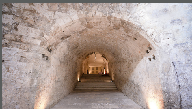
Inside view. Photo taken from the circular vaulted chamber.
