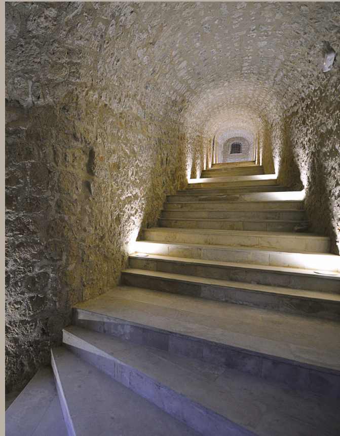
The interior of the sortita to the moat.
