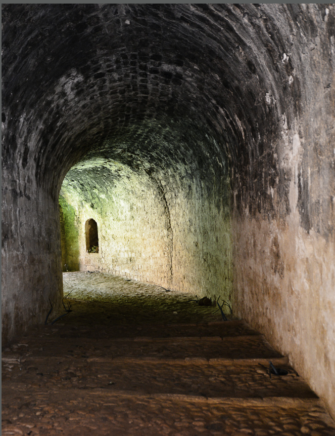
Southern inside view of the vaulted gallery, leading out of the inner city to the exit (at the current KTEL bus terminal)
