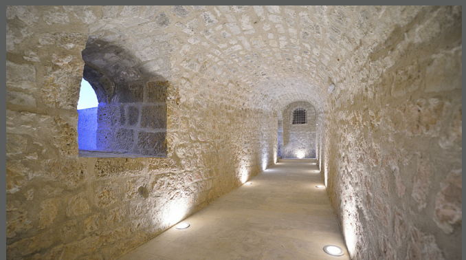
The interior of the sortita leading out the garden theatre “Manos Hatzidakis” to the moat
