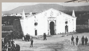
Vitturi Bastion, view from the north; the moat is seen to the left, while the exit of the St. George Gate to the moat is seen to the right. (Photo: G. Gerola)
