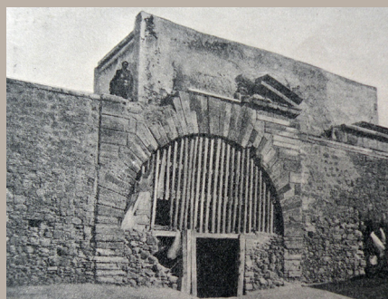
The inside façade of the gate of Dermata, view from southwest. (Photo: G. Gerola).
