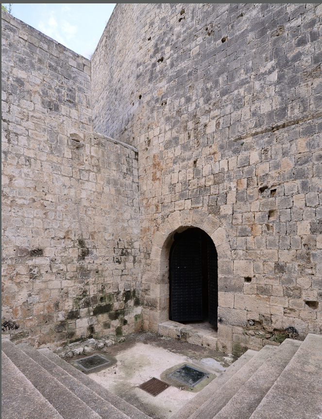
The façade of the outward gallery to the moat.
