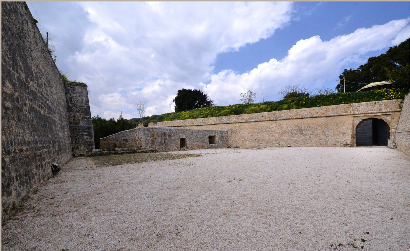
“Low square”, view from the southeast. Two casemates are discernible; the gate leading to the inner city is seen to the right
