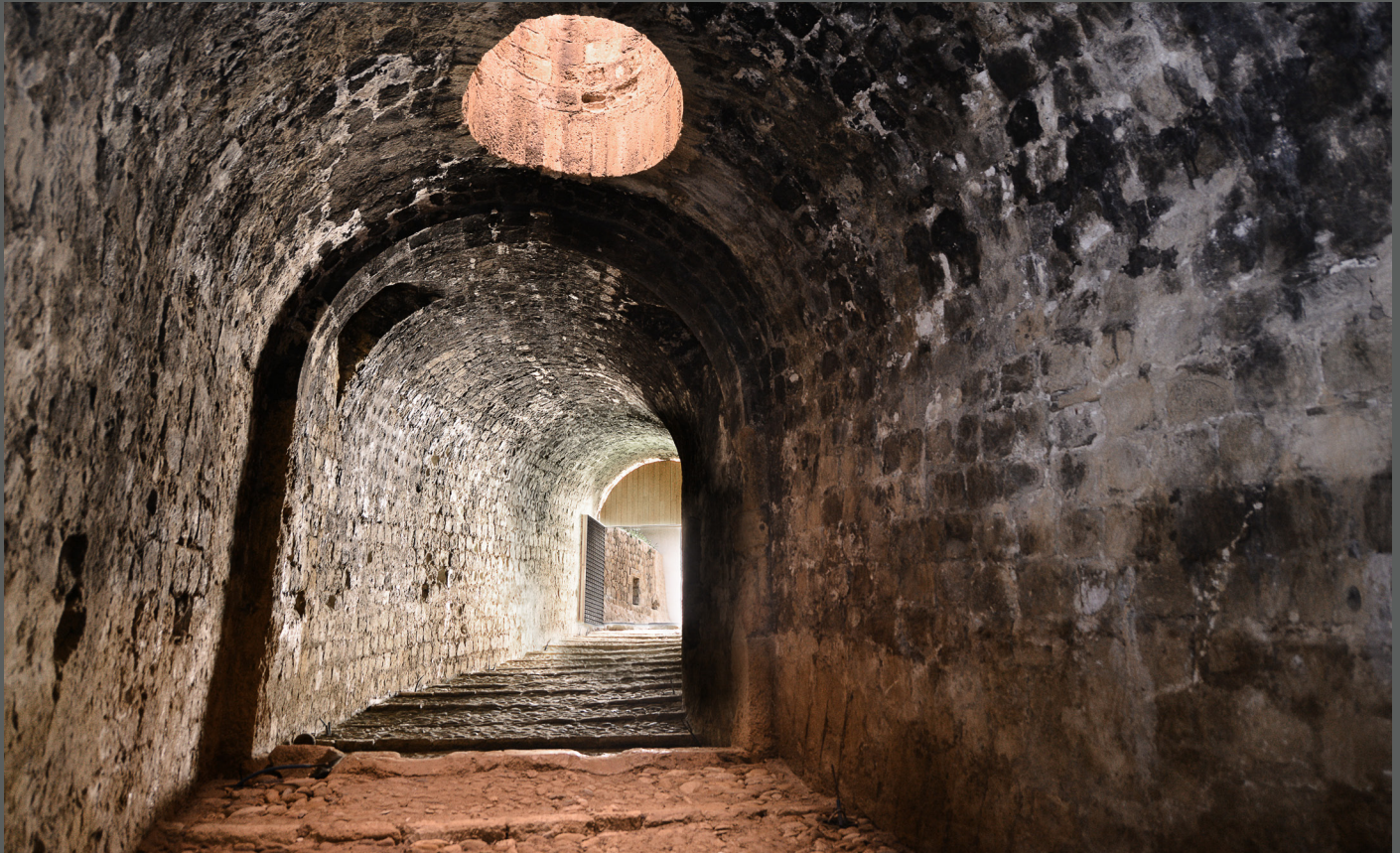
Inside view of the vaulted gallery, leading from the exit (at the current KTEL bus terminal) to the inner city
