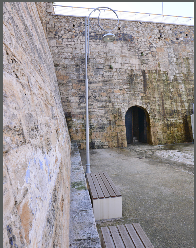
The front face of the exit to the KTEL bus terminal
