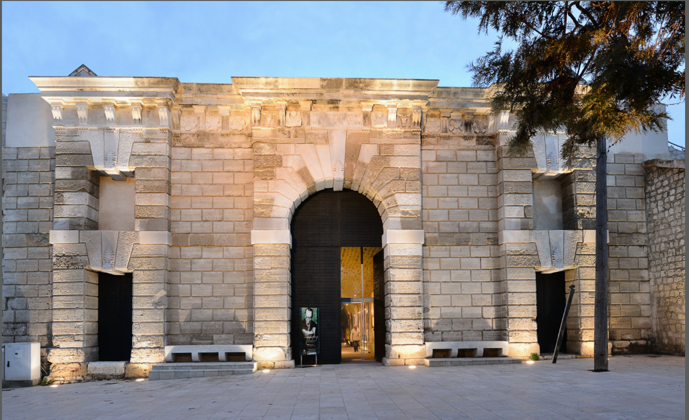
Gate of Jesus view of the inside façade completed in 1587. Influenced by the Renaissance, it bears a Doric-style entablature.
