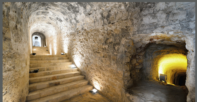
An outward gallery, view from the moat to the low square of the Vitturi Gate. The "mina" (mine) is seen to the right, part of an underground network of tunnels designed for sabotage warfare.
