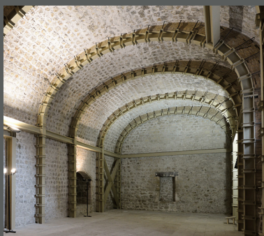
The vaulted chamber inside the gate of Pantocrator, branching off into the galleries leading to the "low square" and the exit out of the city.
