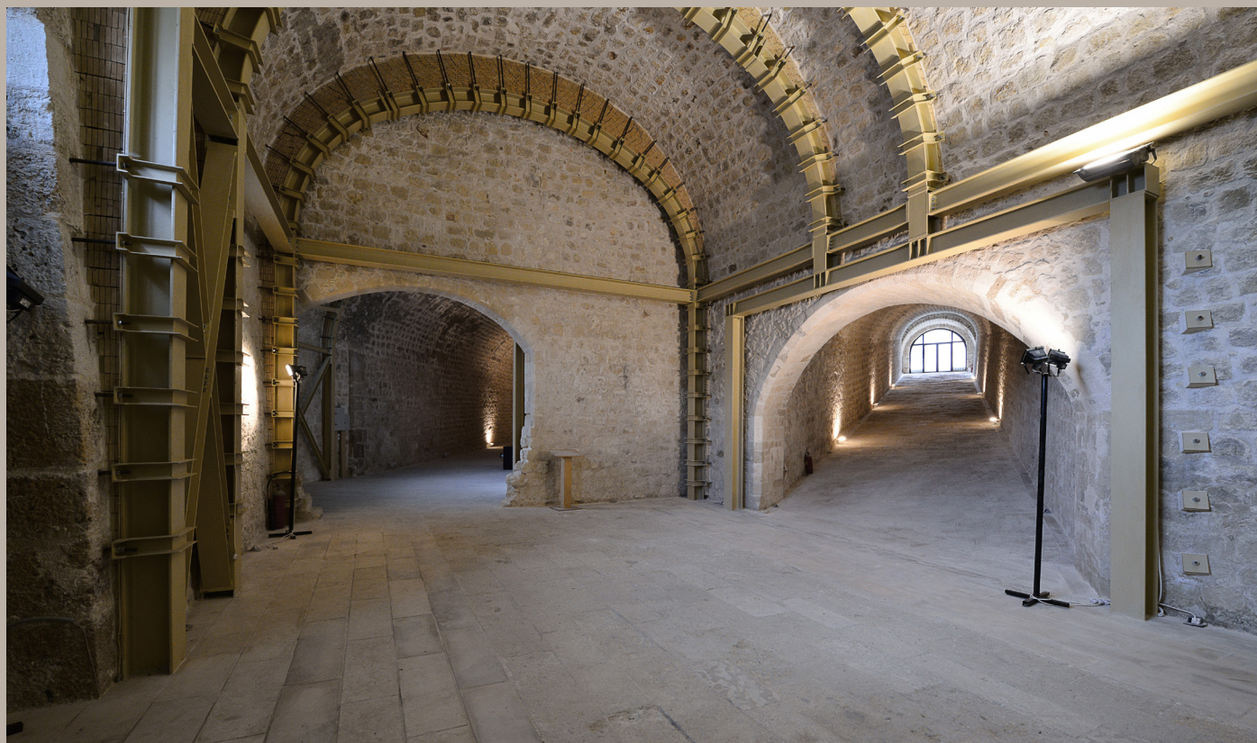
Indoor vaulted chamber of the Pantocrator Gate. To the right, the military use gallery leading to the southern low square; to the left, the public use gallery leading to and from the western suburbs.
