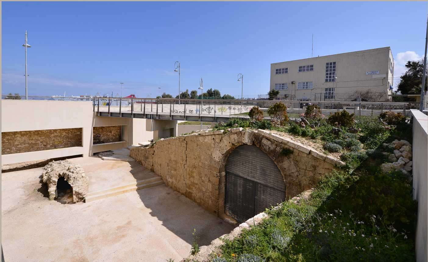
View from Doukos Beaufort street. The gabled façade of the Sabbionara Gate towards the inner city.
