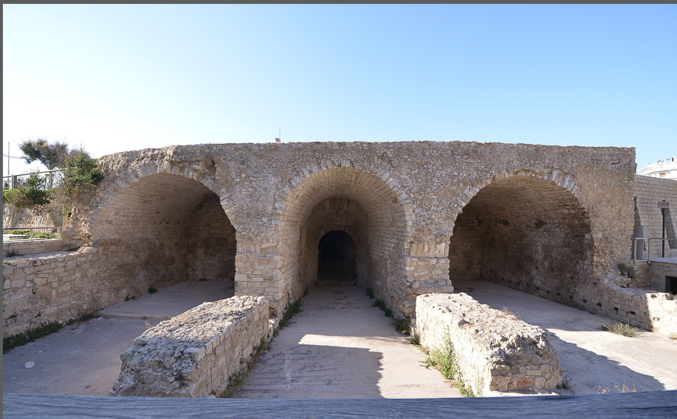
The modern cityward façade of the gate of Dermata. The façade was pulled down to make way for the new road Skordylon. The interior of the gallery is visible, flanked by two vaulted chambers
