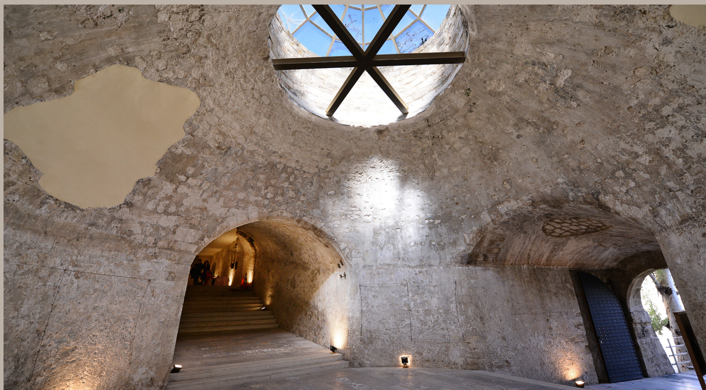
Circular vaulted chamber with lighting and ventilation opening; the exit to the moat (Ikarou Avenue) is seen to the right, while the gallery leading to Eleftheria Square is seen to the left.
