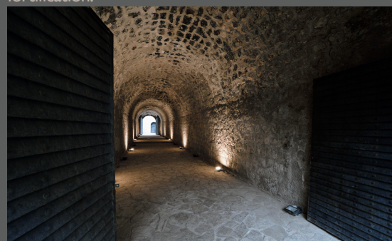
Northern Pantocrator military gate, the interior of the vaulted gallery, a view from the "low square".
