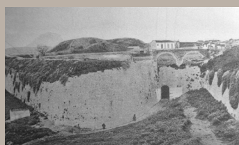
Early 20th century, Gate of St. George, to the inner city. Gabled façade with a central arched gate, flanked by two smaller gates used by the garrison. (Photo: G. Gerola)
