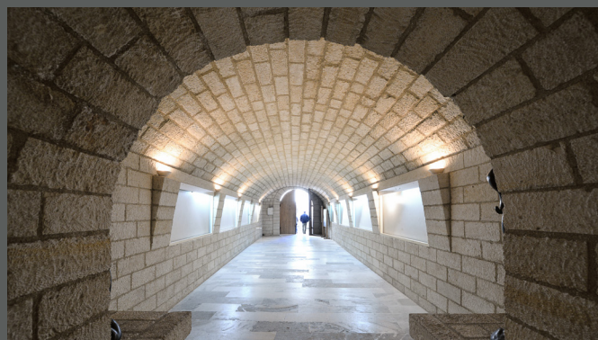
Modern vaulted gallery built to exit the surviving gallery towards Eleftheria Square
